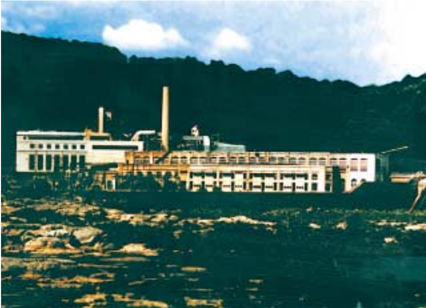
Holtwood Generating Station (See page 4)
