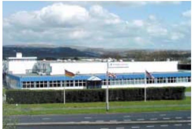
Barden Super Precision Bearing plant located in Plymouth, Devon, U.K.
