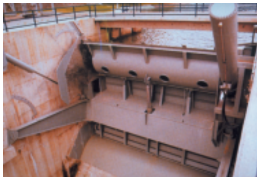
deva.bm®, deva.glide® in hydro engineering: sector weir: regulator flap
