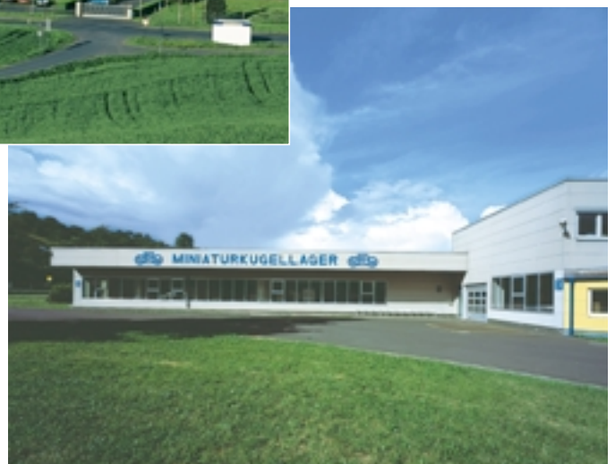
Rimpf production facilities
