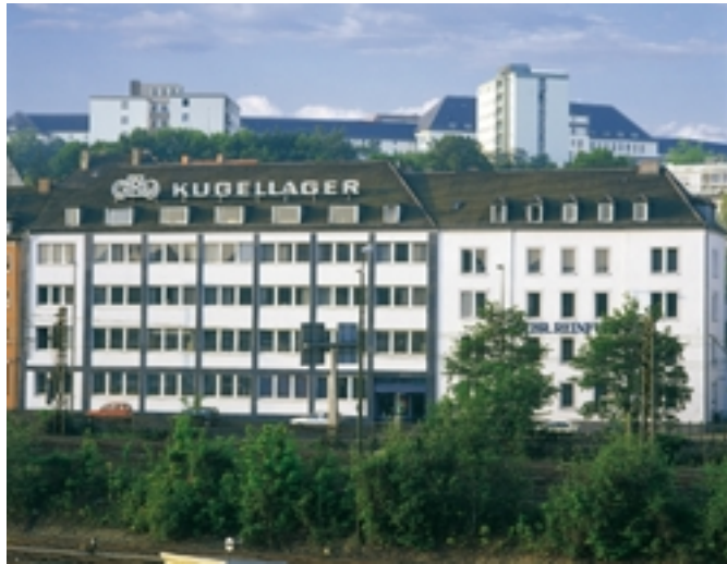
Administration and production facilities in Würzburg
