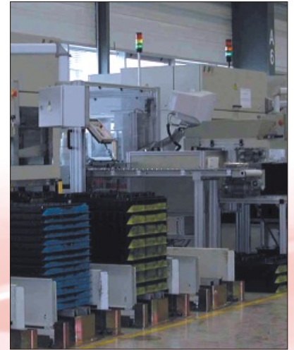
Palettenbefüll -und Abhol- station Pallet filling and destacking station
