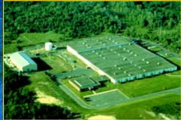
Kop-Flex state-of-the-art manufacturing and service center in Baltimore, MD
