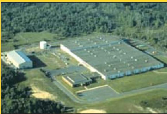
KOP-FLEX's state-of-the-art Manufacturing and Service Center in Baltimore, MD
