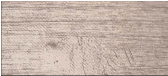
Wear caused by static vibration
