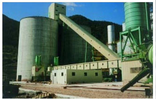
Rex AFT pan conveyor installation.
