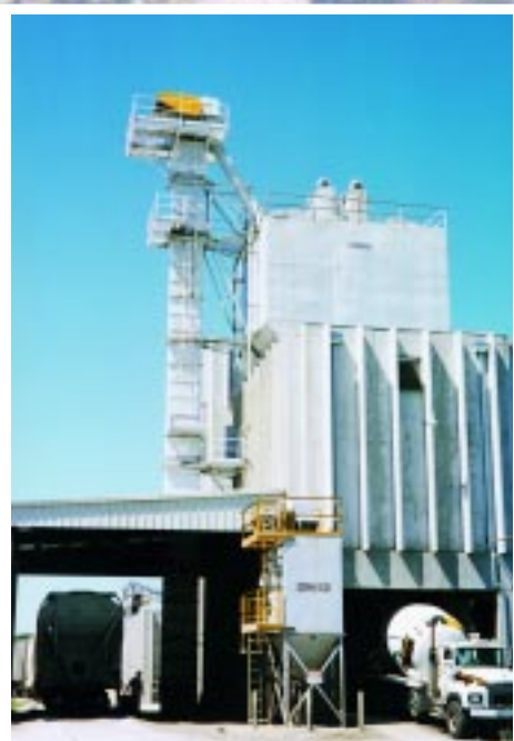
Rex bucket elevator at cement terminal.
