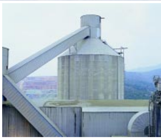
Rex AFT pan conveyors handling cement clinker.
