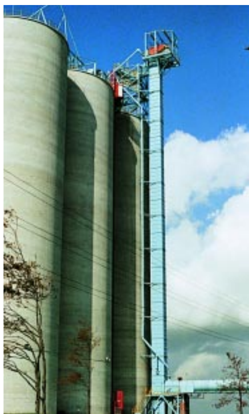
Rex belt bucket elevator handling finish cement.
