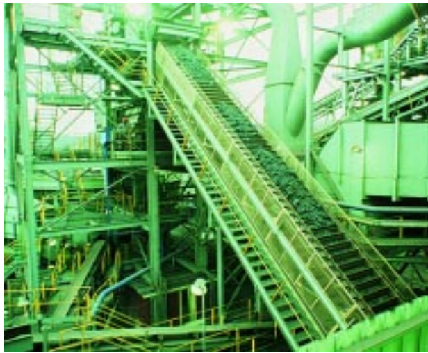
Rex Style C pan conveyor handling hot steel sinter.
