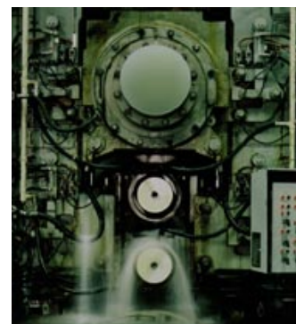
Steel rolling mill
