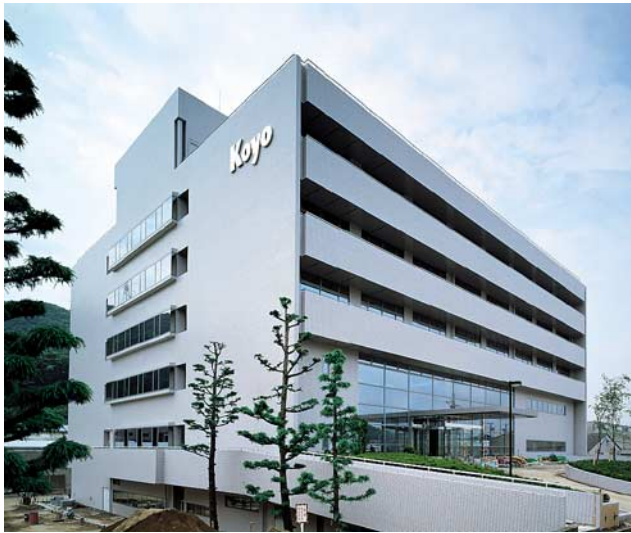
Technical Center (Osaka, Japan)
